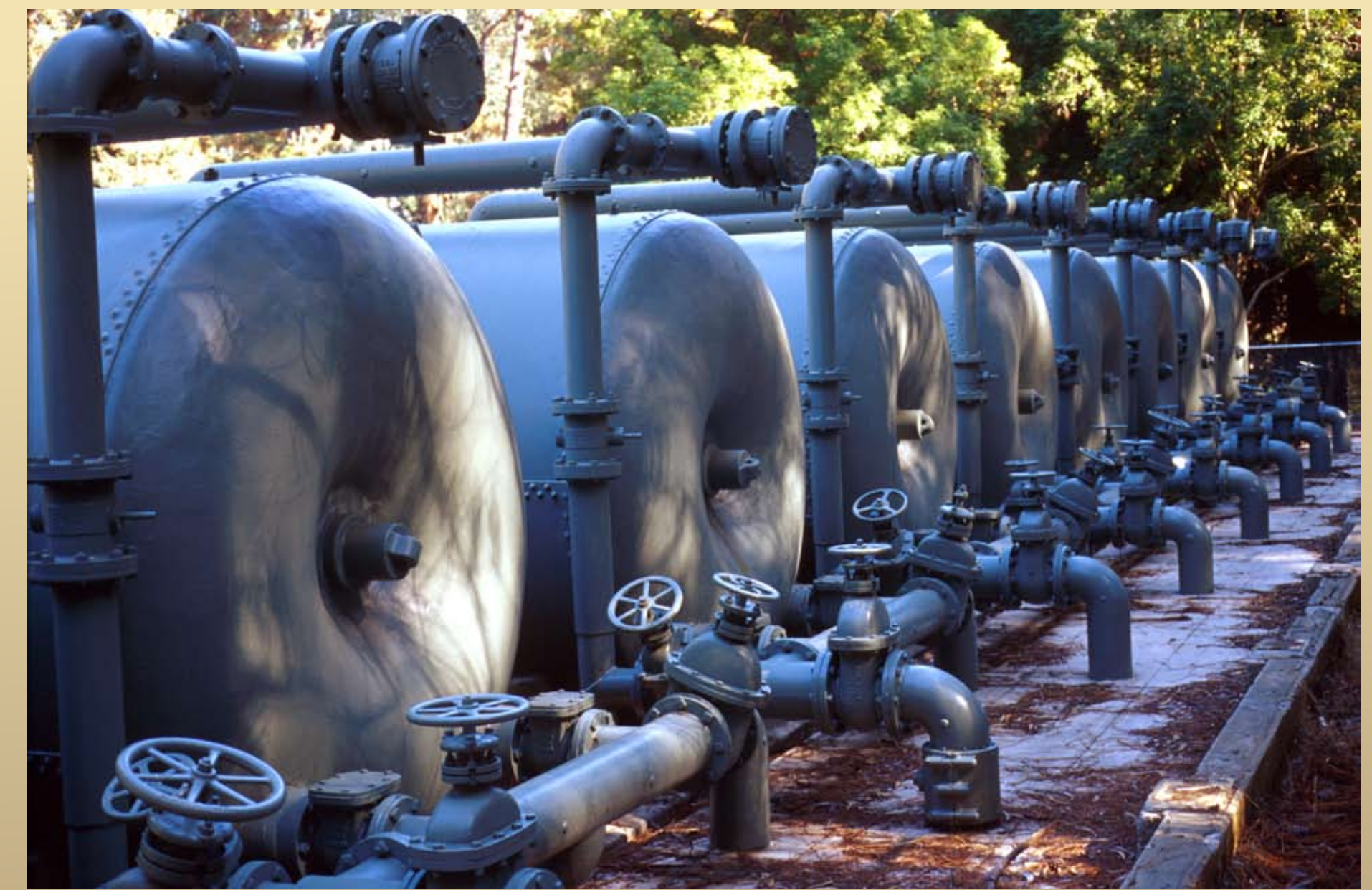
Water was forced through the sand contained in these drums in order to filter out impurities.
